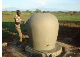
Lime added to the final layer of plastering makes the tank light grey and keeps it cooler.
