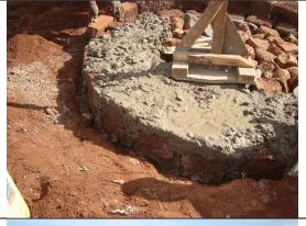
And tramp the mortar to gaps by a self-made tool as shown in the picture.
