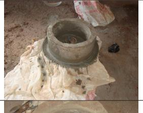
When the cement ring has dried make the second part of the lid. This is the cement plate that forms the actual lid for the mouth of the tank.
