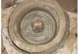
Use a tin in the middle to keep it open. This is where the water passes through to the tank.
