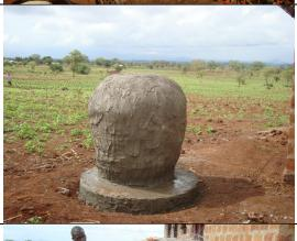
Plaster for the first time. Use a mixture of 1 : 2 (cement : sand). Make a layer of about half an inch or one inch towards the bottom.
